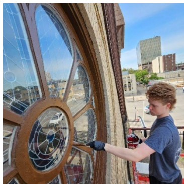
Eli applying putty/wood filler, then epoxy, then paint.
