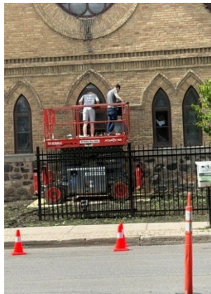
Positioning the scissor lift on the west side.
